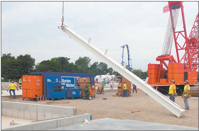
The first of 299 columns being laid at FCA's paint shop building.
