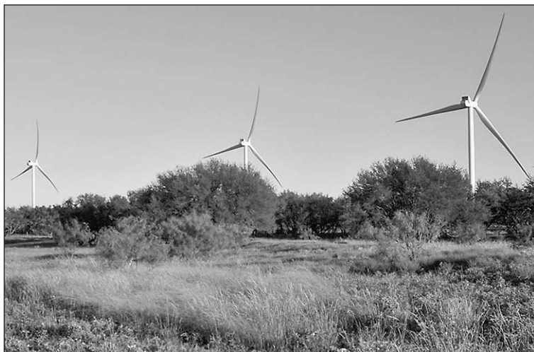
Wind turbines power the GM Arlington, Texas, Assembly Plant.
