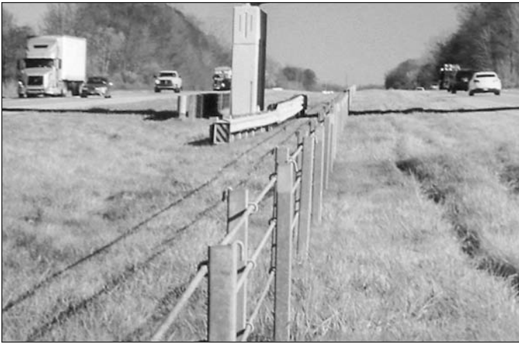
Cable barriers can stop crashing cars from crossing medians.
