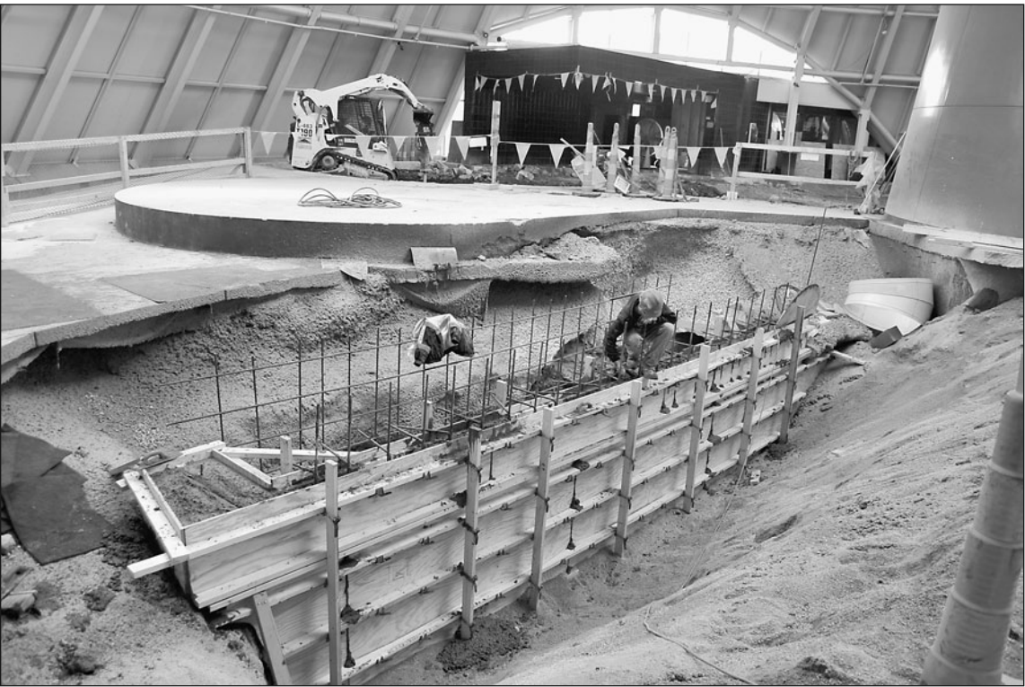
Work began immediately to fill the sink hole and repair the damage it caused at the Corvette museum.
