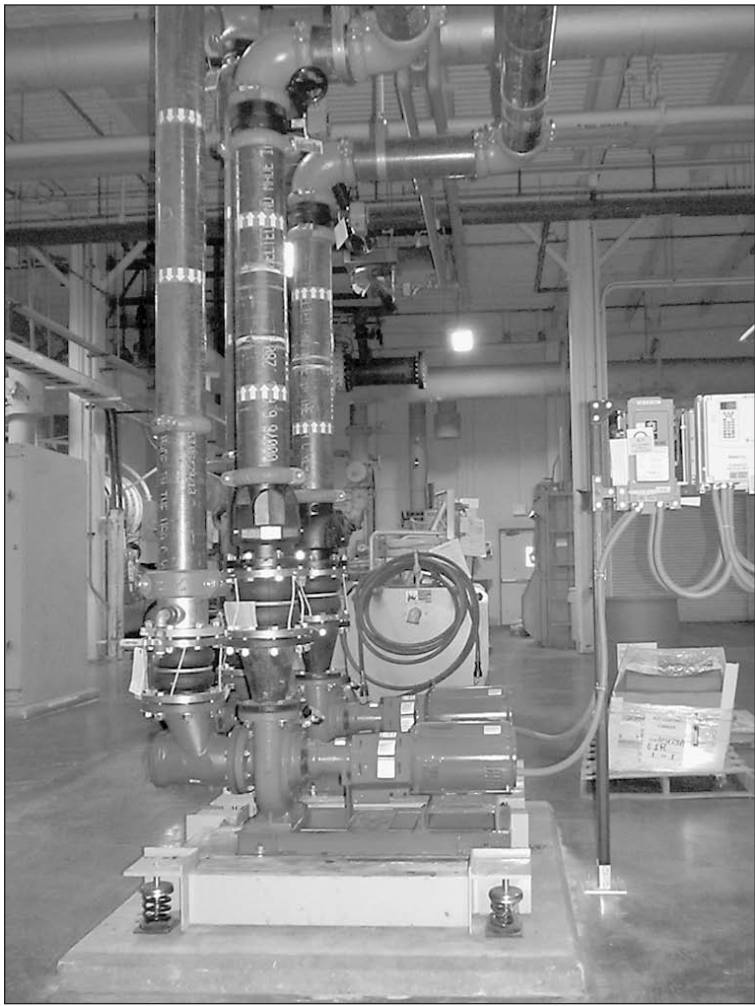
GM's Kokomo pumps capture heat to warm water for manufacturing.
