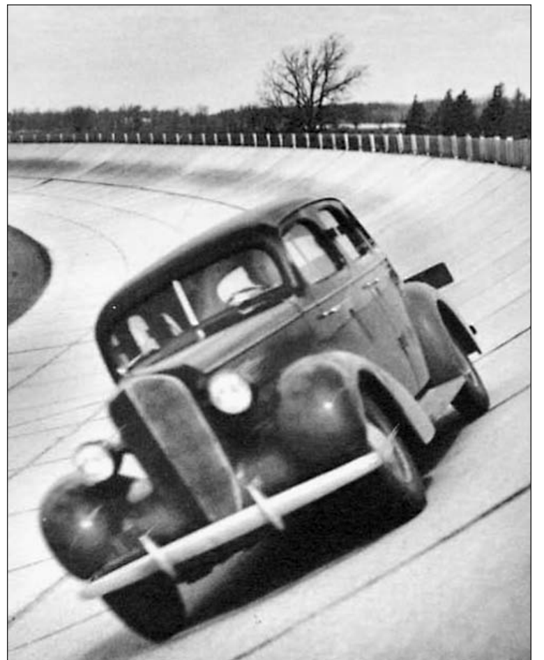
Then-new 1937 Chevrolet gets tested at GM's Milford Proving Ground.
