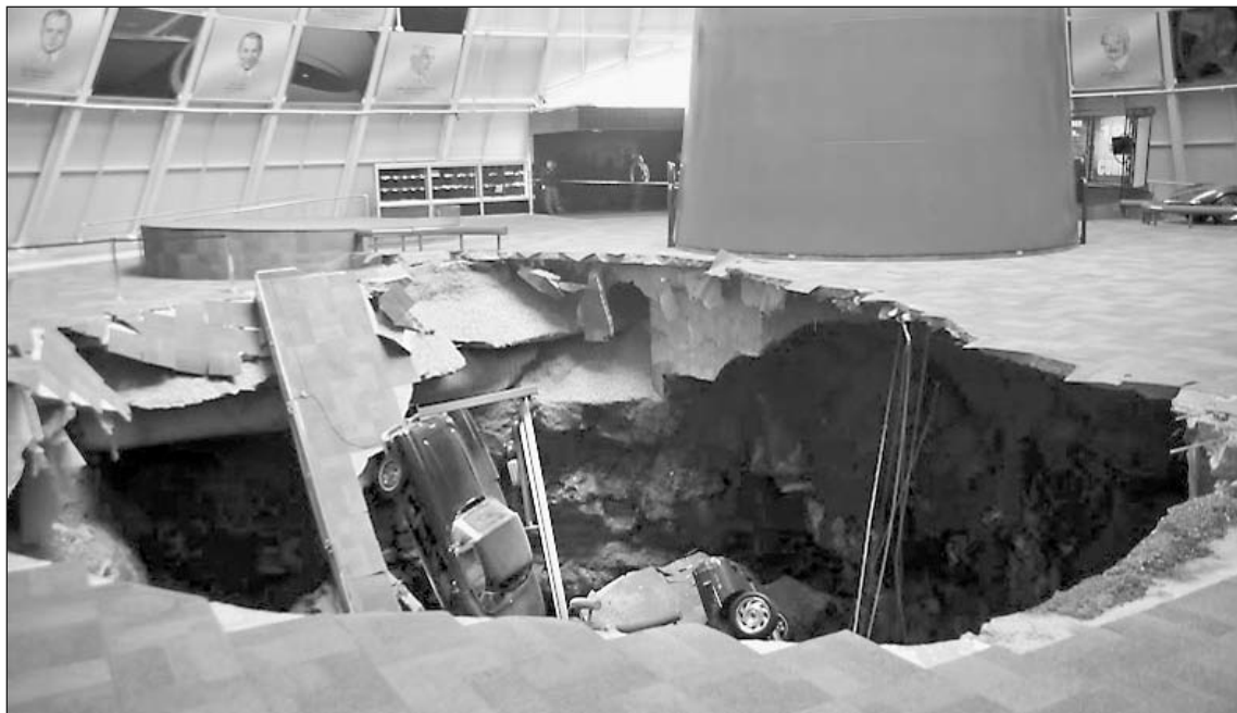
Eight Corvettes – two from GM Heritage Center – fell 30 feet when a sinkhole opened at the Corvette Museum.
