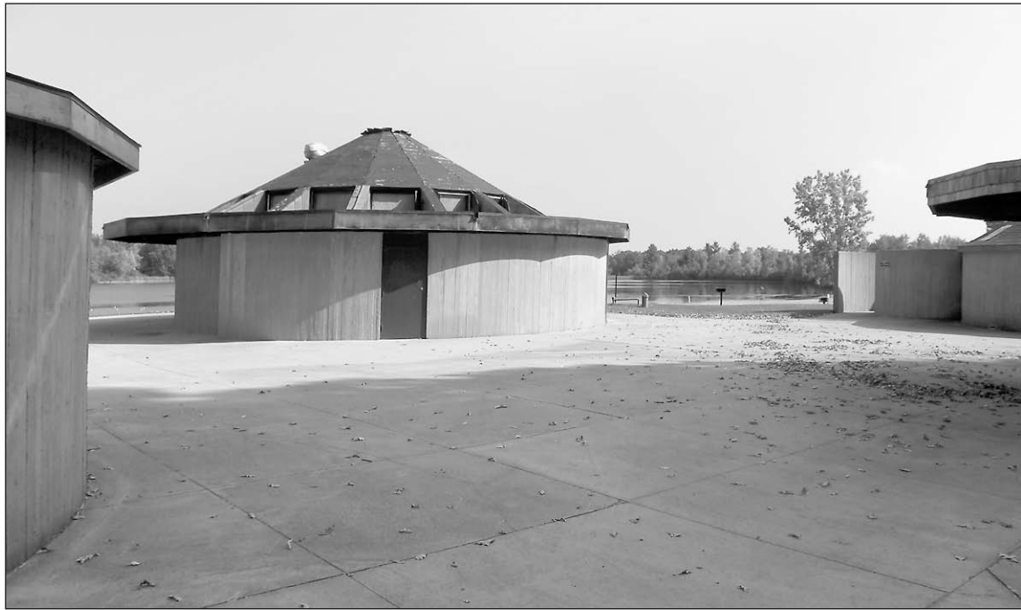
The Lower Trout Lake Bathhouse Complex and Contact Station in the Bald Mountain Recreation Area.
