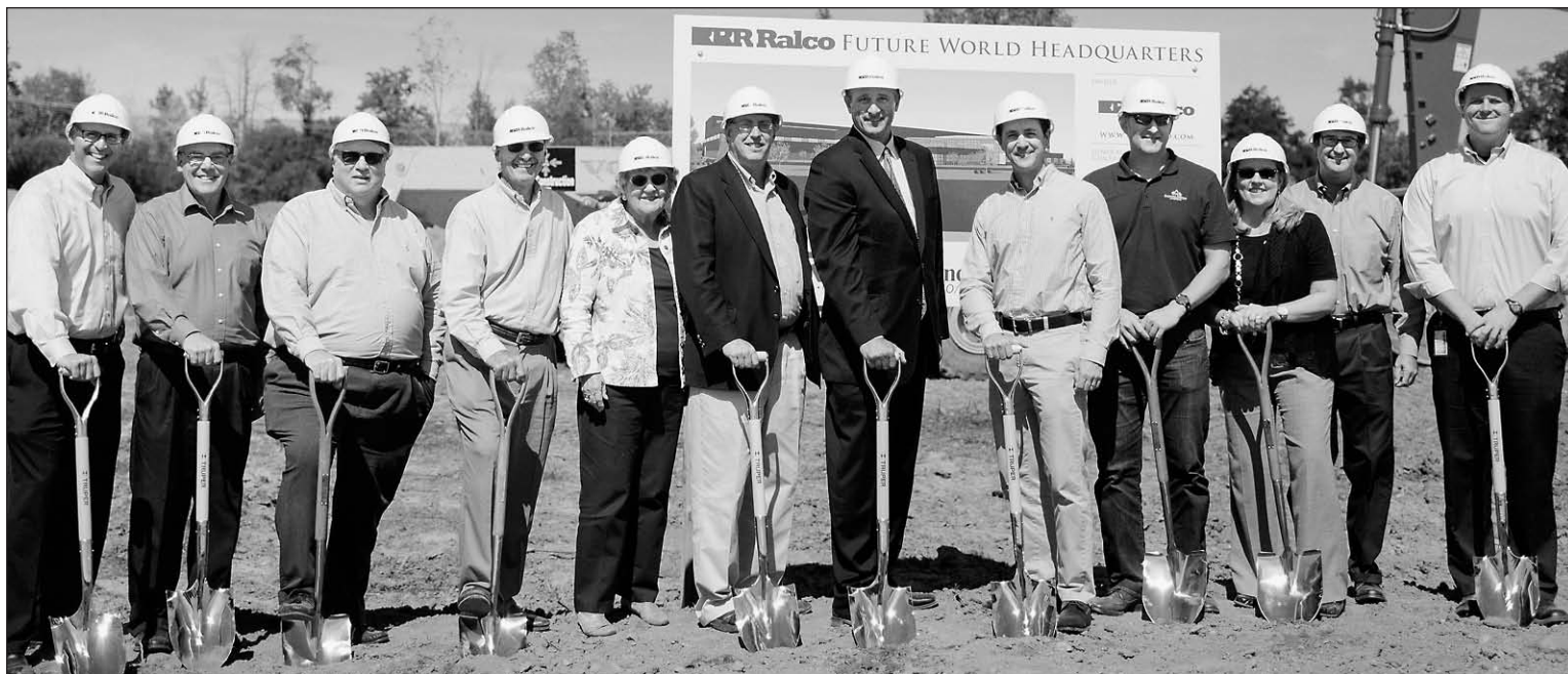
Officials from the Auburn Hills government and Ralco Industries recently broke ground on a new world headquarters for the auto supplier.
