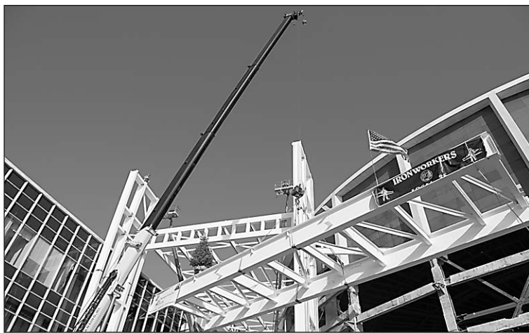
Cobo Center is getting a new glass atrium.
