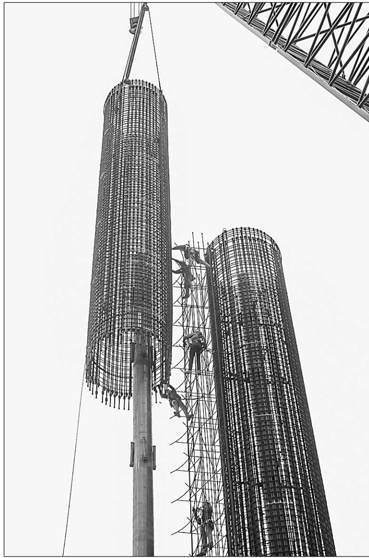
Joseph A. Blum photo of construction of the San Francisco-Oakland Bay Bridge. Photos courtesy Macomb Community College
