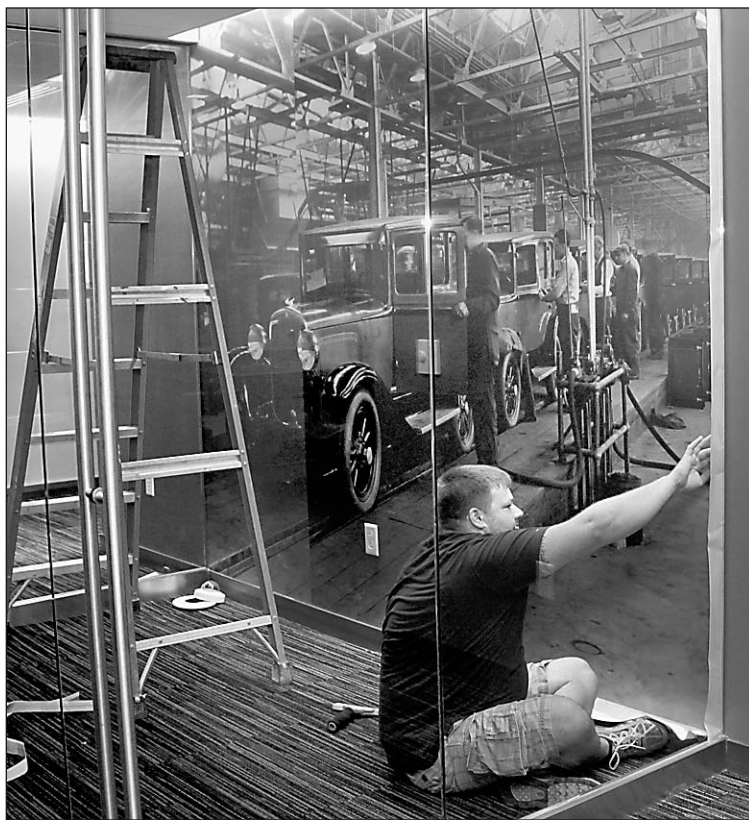
A worker installs a mural featuring vintage Chrysler photography.
